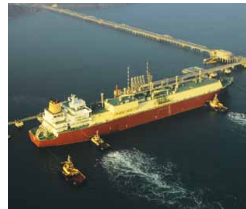
Fully-commissioned in 2010, South Hook is one of the biggest and most advanced LNG terminals in the world.
